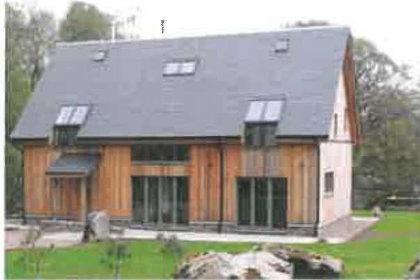
Figure 15 – Greenwood House, Pyatshaw: Timber-clad approach
